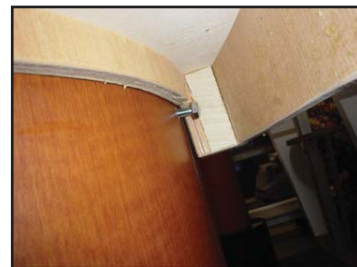
Attach Front Counter Top using Thumbscrews.
