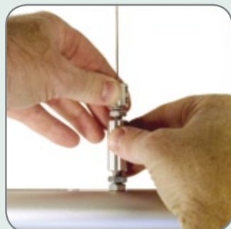
Attach and tension the wire and Turnbuckle top nut on the assembly
