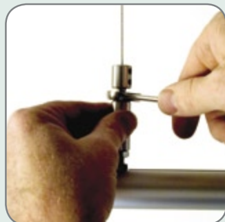
Complete the assembly by tightening both jam nuts on the Turnbuckle
