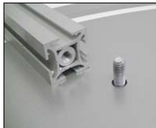
Base Plate Connection
